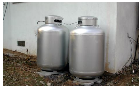
Correctly stored compressed gas: upright, secured with safety caps in place and off wet ground to prevent corrosion.
