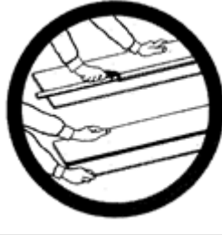
Cutting asbestos-containing wall board by hand.
