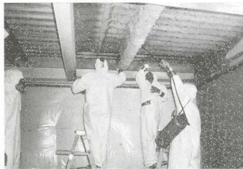
Typical high risk abatement project
